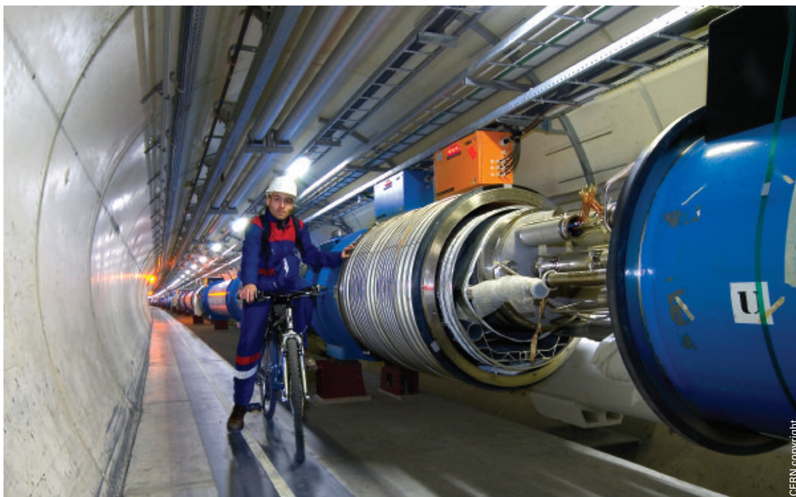
A technician cycles to work in the LHC tunnel. This photograph was taken during the installation of the superconducting solenoids; two of the metal tubes will carry the proton beams
